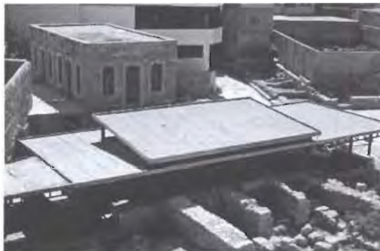
Madaba: shelter over the Burnt Palace
