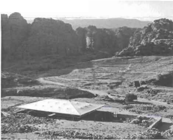
Petra, Petra Church, the space frame shelter
