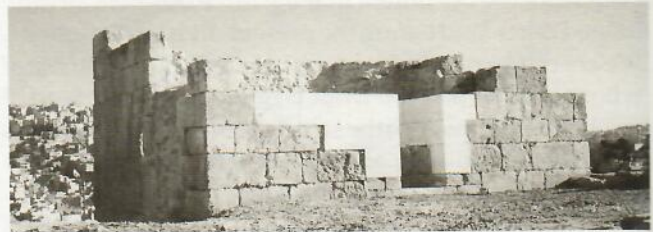
The north side of the tower after restoration. The new stones are the same limestone as the ancient ones. They will weather from white to soft pink in about 10 years.
