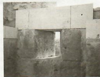
Restored arrow slit
