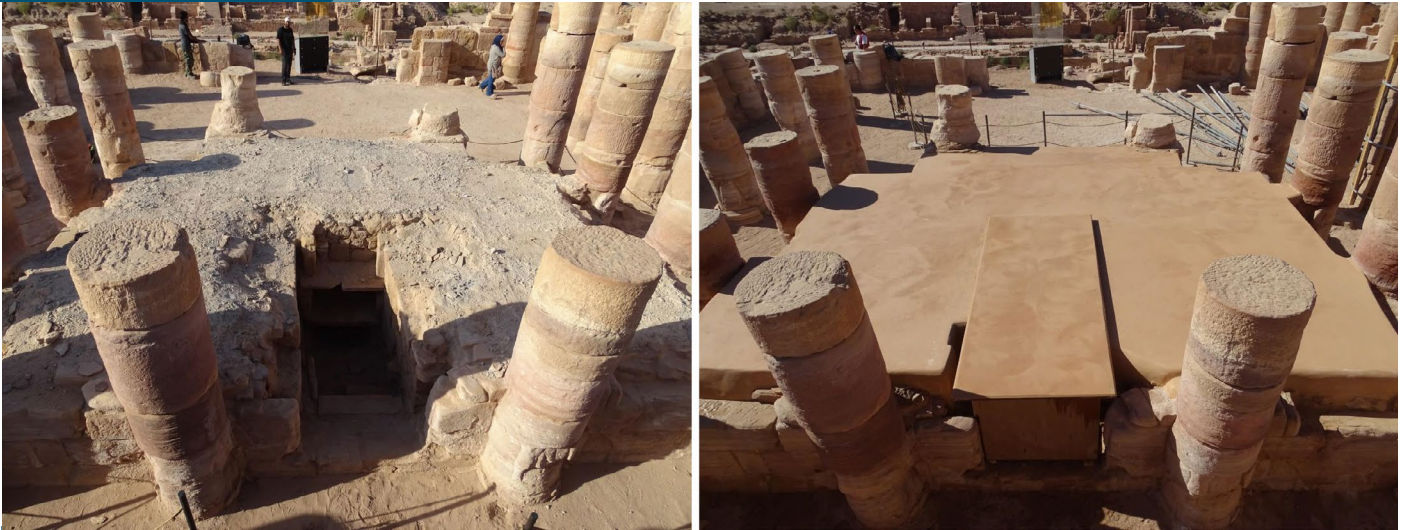
Fig. 81. The cella podium within the Temple before and after the application of a protective mortar capping (photos by Franco Sciorilli)
